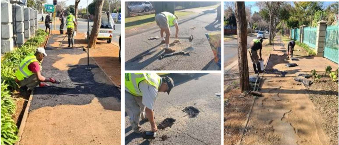
Pothole Restoring Team more than 150 potholes & many crack fillings
